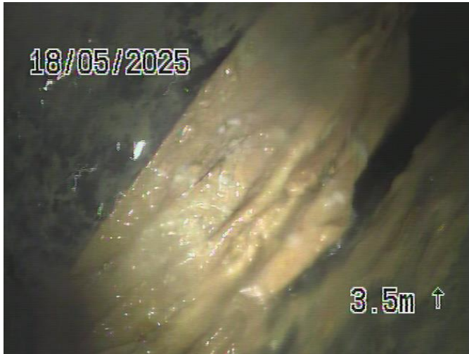
Picture of blockage where you can see Wet wipes getting stuck in the stack
